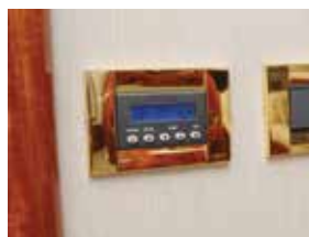
The Qht keypad/display is available with a variety of decorative bezels to complement any interior
